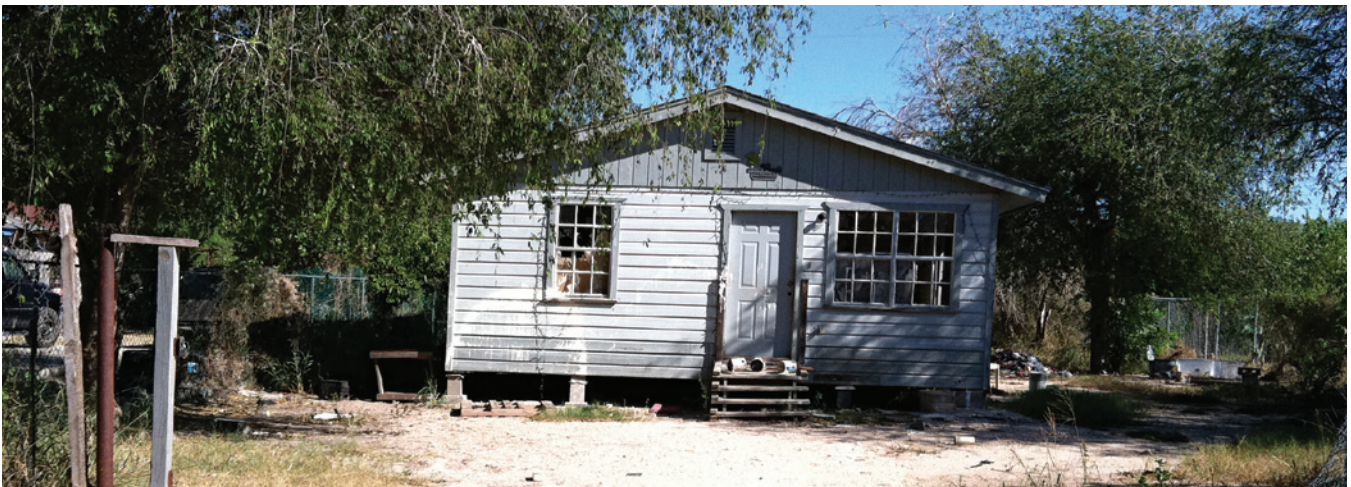
Colonias often lack basics such as heat and electricity.
